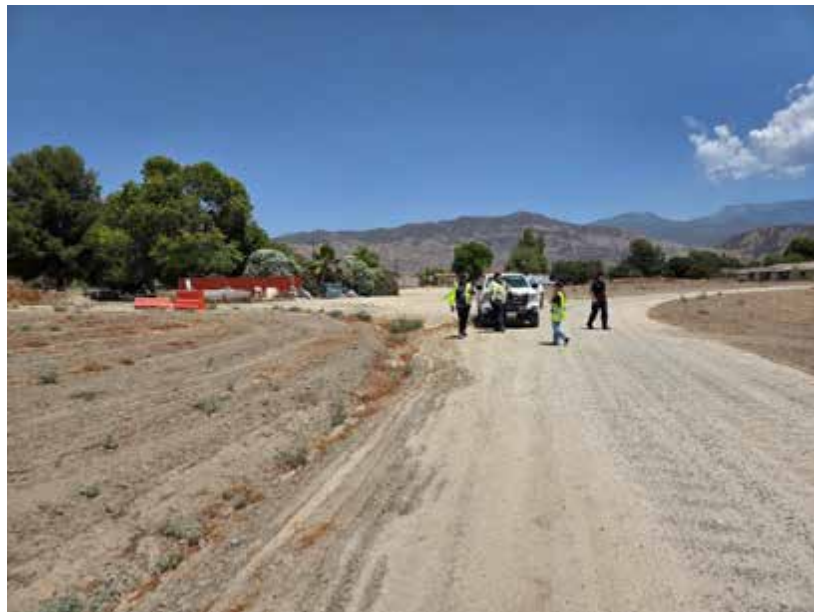
Looking northeast along the Line J alignment towards the beginning of the line (the drop inlet and basin)
