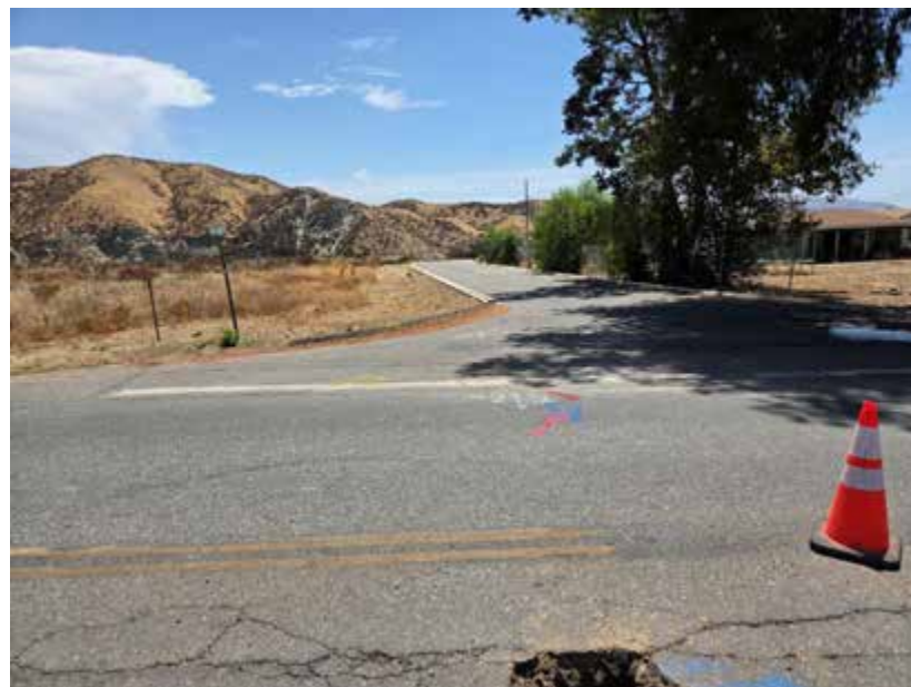
Looking south (and downgradient) at Castile Canyon Road along the Line J alignment as it turns toward Poppet Flats Road.
