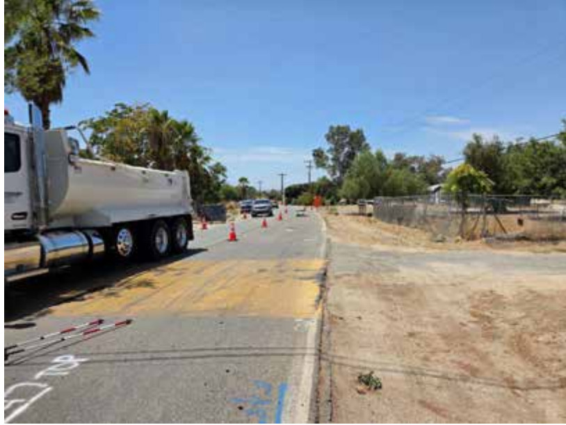
Looking west at Castile Canyon Road along the Line J alignment
